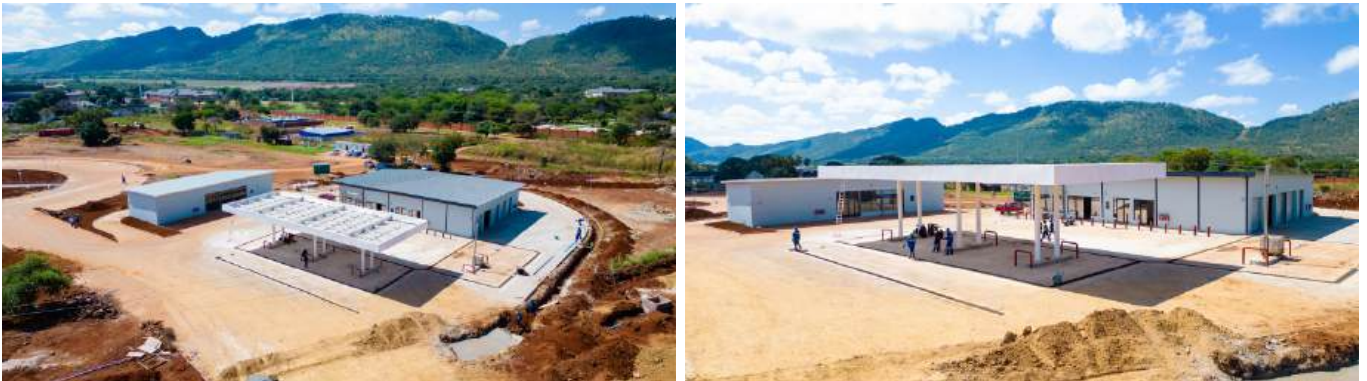
Figure 2: Service Station Forecourt and convenience store structure
